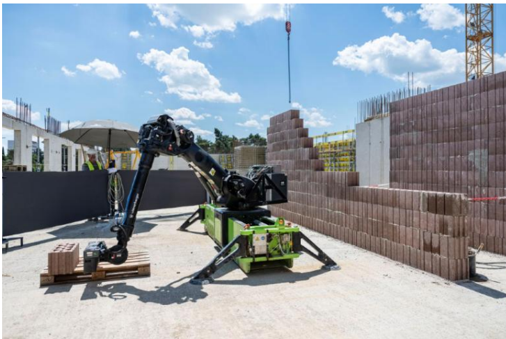
Walter can lift bricks weighing up to 52 kg © PORR/Jan Hrdý
